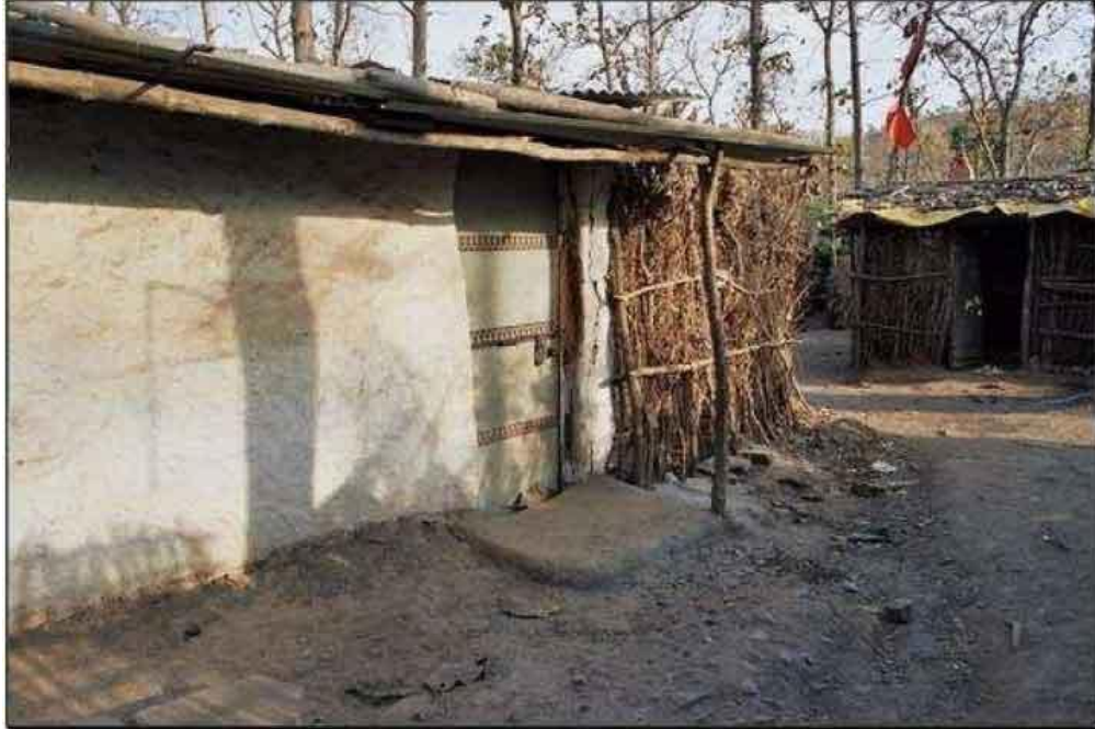
Fig. 92: Lane and houses of the district of Dukhia. The house of left is built in cob with a sheet roof. The house of right-hand side is made up of branches and a roof of branches waterproofed by a cover. Source: CREMIN Emilie, March 2005.
