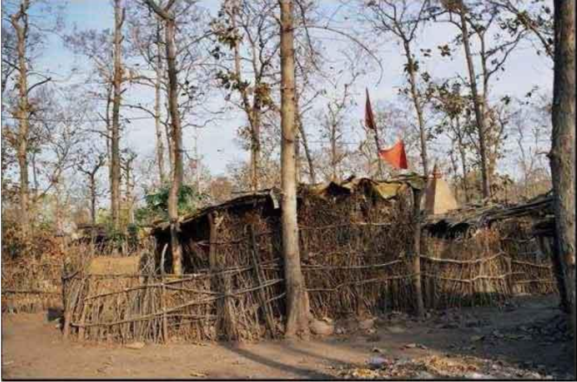
Fig. 93: House belonging to a sâdhu, remarkable by the triangular orange flags. Opposite, a cattle shed lodges some sacred cows. On the right-hand side, the hut of a sâdhu. The walls are composed of branches while the roof is composed of a structure of wood, cover of a cover retained by stones. Source: CREMIN Emilie, March 2005.
