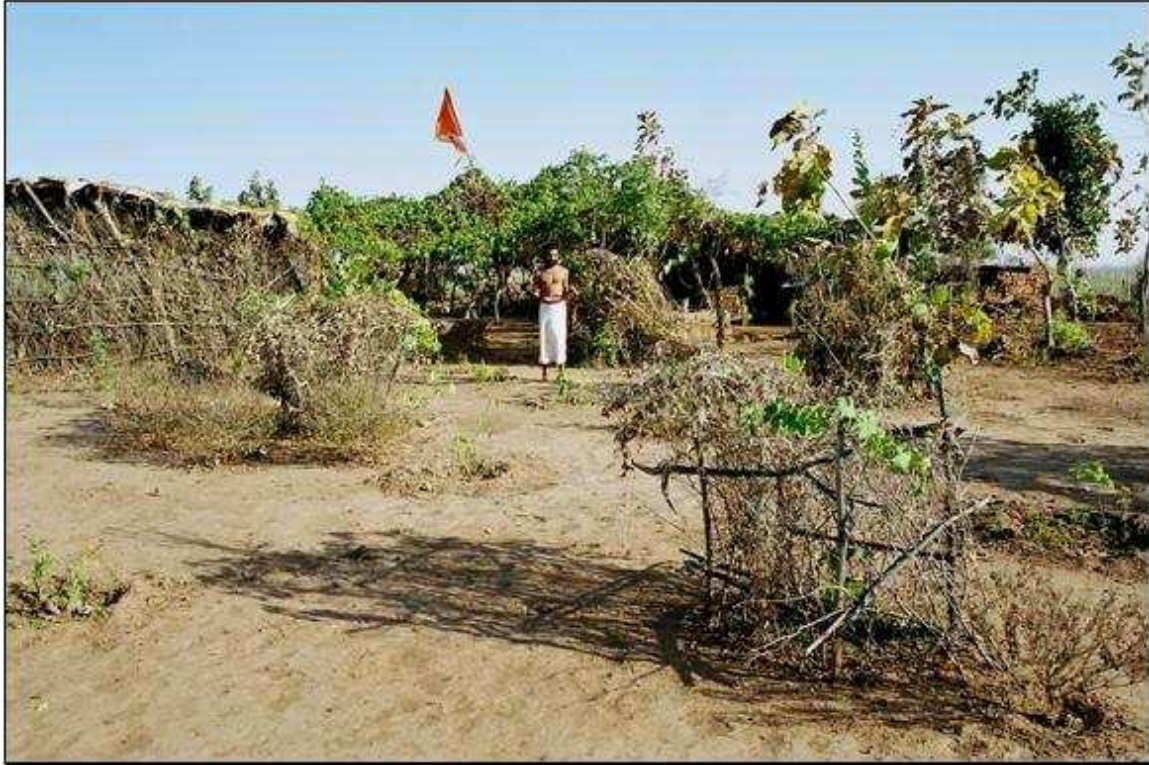
Fig. 66: Hut of a sâdhu, called the “OM Shanti Ashram,” standing insulated on the top of the island. This dwelling is built in the whole out of vegetable materials, with the climbing plants covering the part where the fire is located. Only the part being used as shelter is built out of brick and is covered with a sheet roof. Around, a kitchen garden allows the sâdhu and his disciples to be partially self-sufficient in food. Source: CREMIN Emilie, January 2005.
